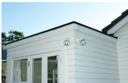
Figure 4: Bitumen membrane skillion roof
