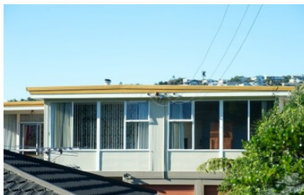
Figure 3: Very low pitched roof
